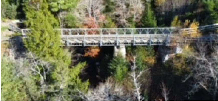
McKeen Brook Bridge in Aspen
